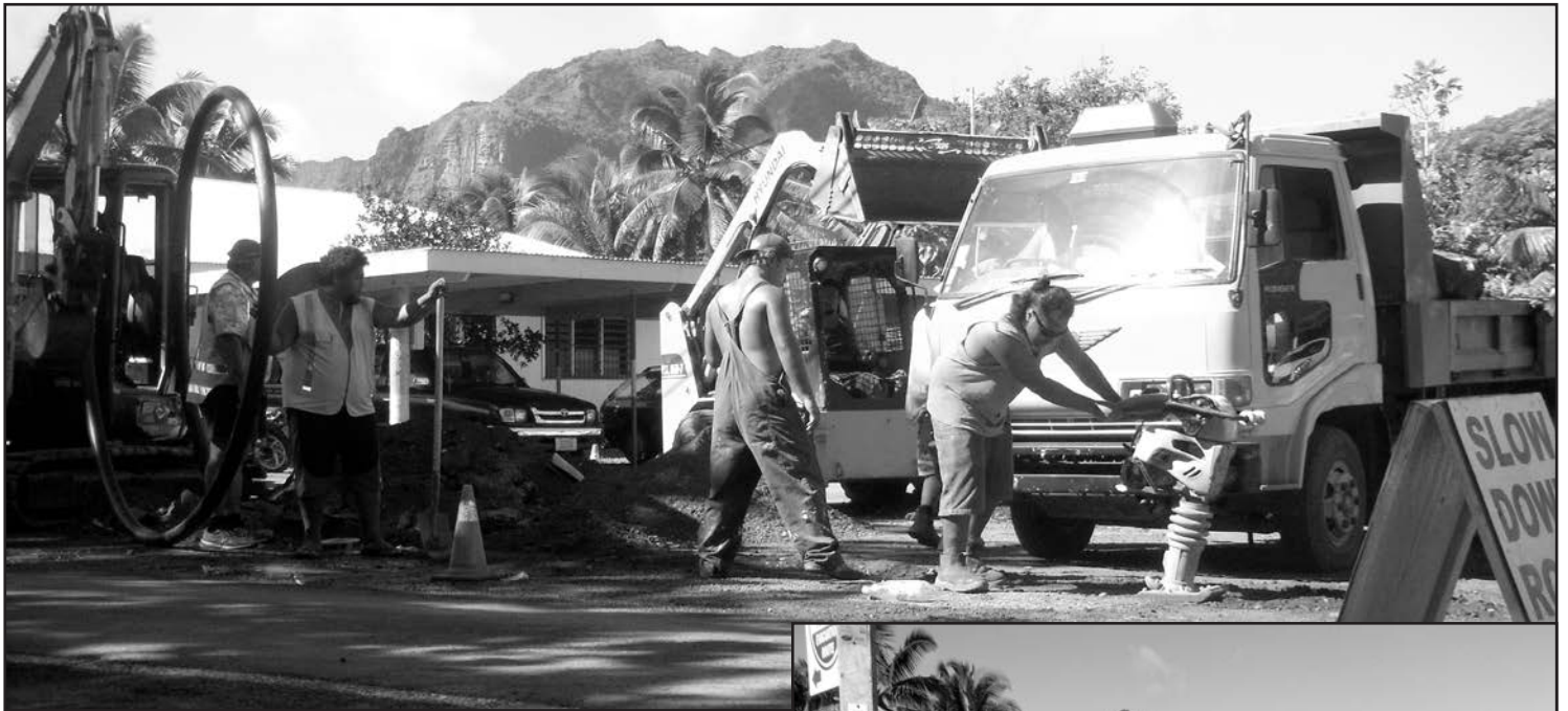
Above: Laying sub-main water pipes outside Motor Centre, Panama
